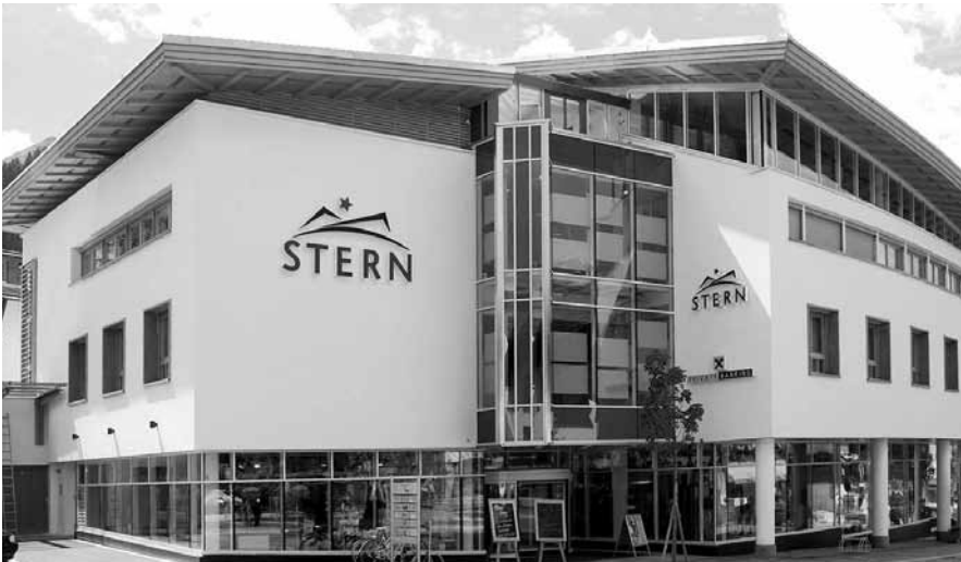
STERN-Passage in Riezlern
